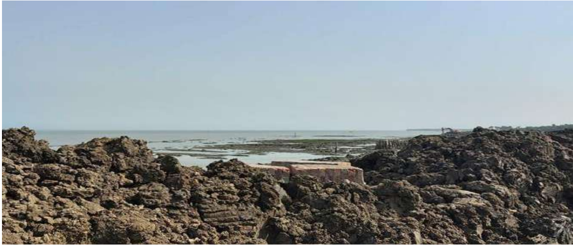
Figure 18 Degraded coastline in Sagar Island
